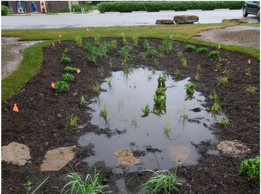
This photo is a rain garden planted next to a parking lot about eight hours after a rainstorm. Notice how the deepest water remains in the center but the edges of the garden are already drying out.
